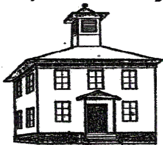
Graded School - 1869 Richford, N.Y.
